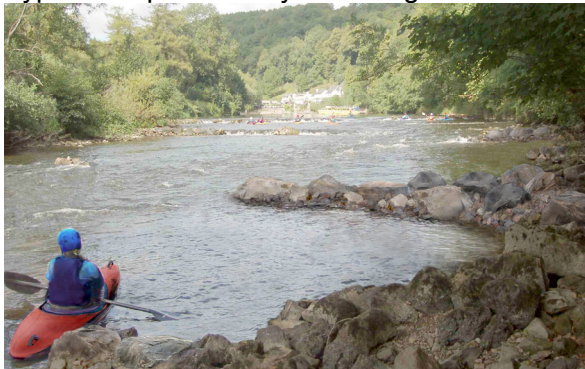
Typical Proposed Groyne Arrangement
